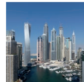
DUBAI Saving energy in air conditioning systems
